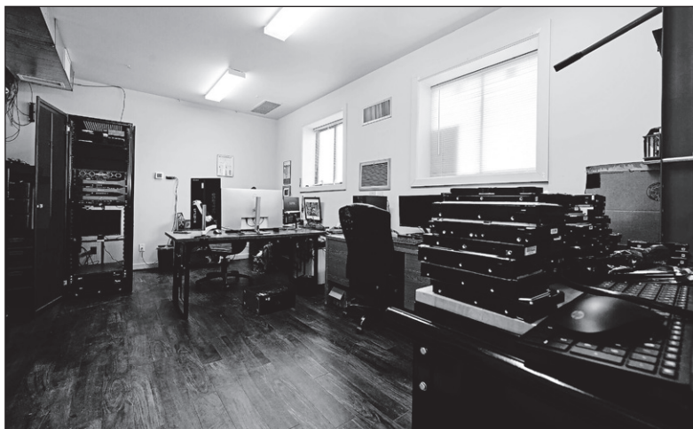
The Interior at Tri-Tech (above) and the server room (below).
